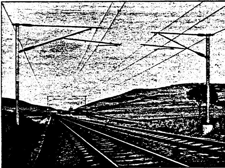
A computer-based system developed by BREL is used extensively by Balfour Beatty to simulate a variety of overhead electrification equipment for contracts through the world.
